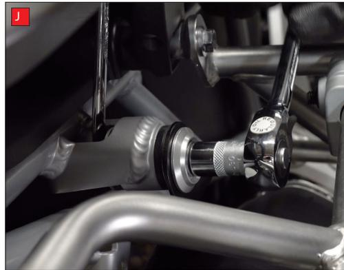
I) Fully tighten the 2 bolts on the back of the silencer mounting bracket.
